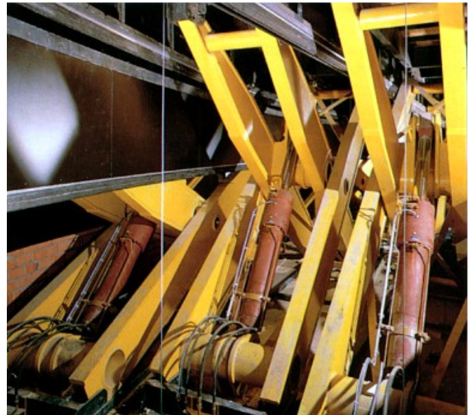
Ratchetless holding of the stage-position in case of a failure of the hydraulic system.
