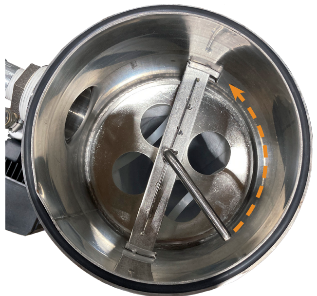
Loosening the filter pressure clamp
